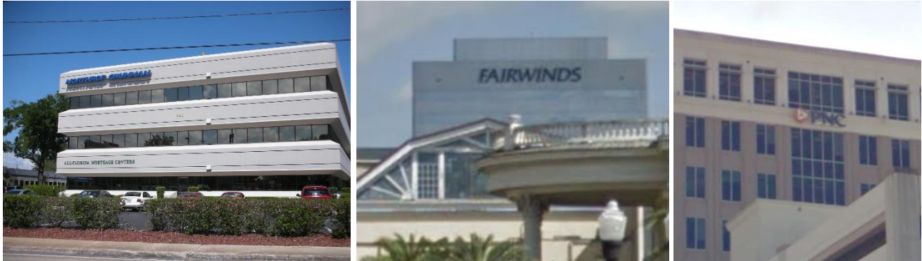
Figure 49. Wall Sign Above Second Story
