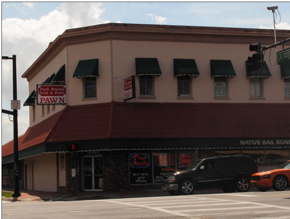
Figure 5: Building Frontage and Architecture
